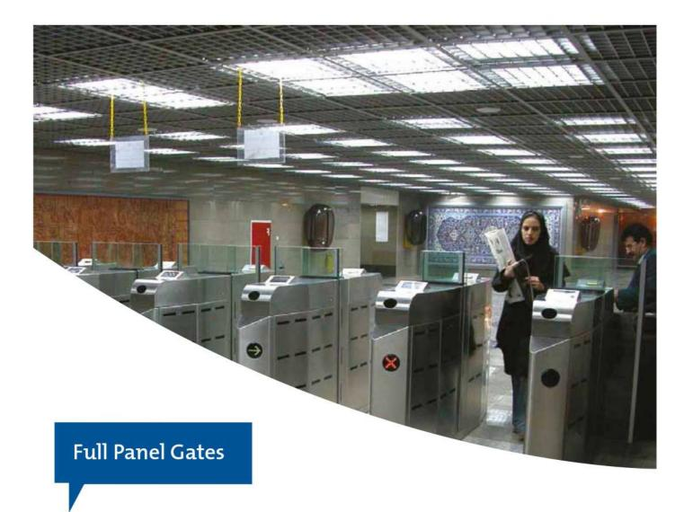
The Full Panel Gate offers high security prevention through the use of tall retractable glass panels which slide into the cabinet when the passenger's ticket is authorised.
